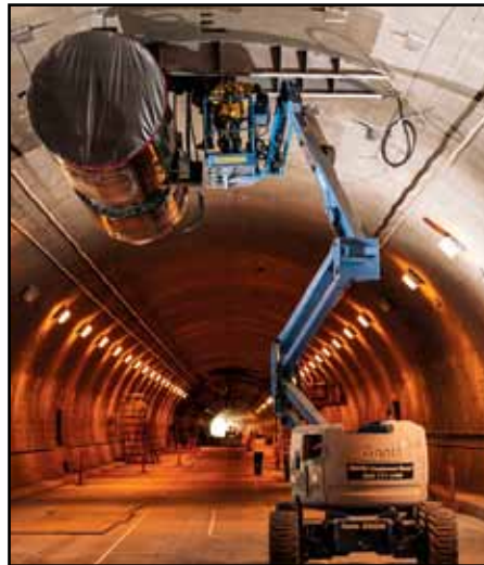
Jet fans are part of the Caldecott Tunnel's state of the art system of fire and life safety. In the far left photo, a 200 horsepower jet fan is delivered to the east portal of the fourth bore. The middle photo shows one of the 19 jets being carefully placed along the tunnel roof, and the far right photo shows workman laboring on the permanent soundwall on the western side. PHOTOS BY KARL NIELSEN, MTC
