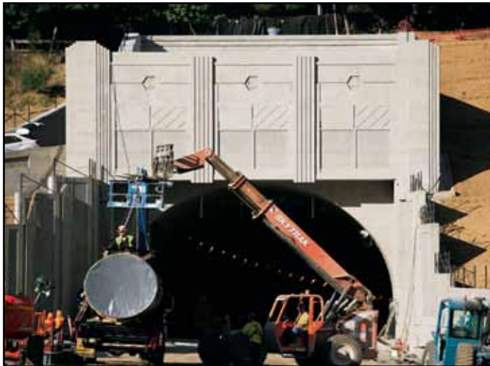
Jet fans are part of the Caldecott Tunnel's state of the art system of fire and life safety. In the far left photo, a 200 horsepower jet fan is delivered to the east portal of the fourth bore. The middle photo shows one of the 19 jets being carefully placed along the tunnel roof, and the far right photo shows workman laboring on the permanent soundwall on the western side. PHOTOS BY KARL NIELSEN, MTC
