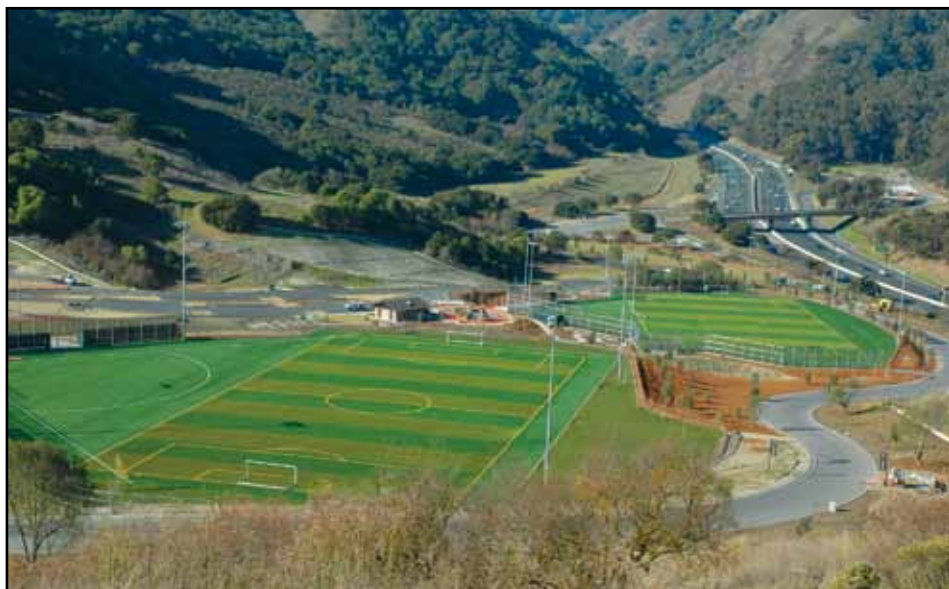
Field #1 (upper right) may be available in early spring. Field #2 (lower left) still needs an access road and parking lot completed.
