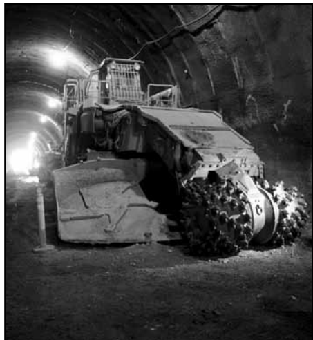
COURTESY OF CALTRANS, DIST 4, JOHN HUSEBY PHOTOGRAPHER
