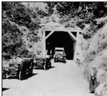
Original Kennedy/Broadway Tunnel above current Caldecott Tunnel.
